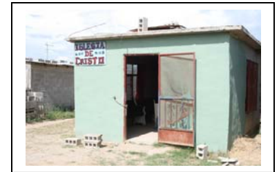
The 5 de Mayo church building
